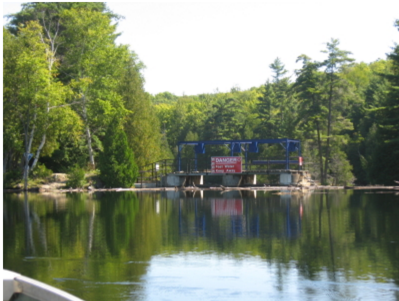
The Dam: August 2008 Photograph by the author
