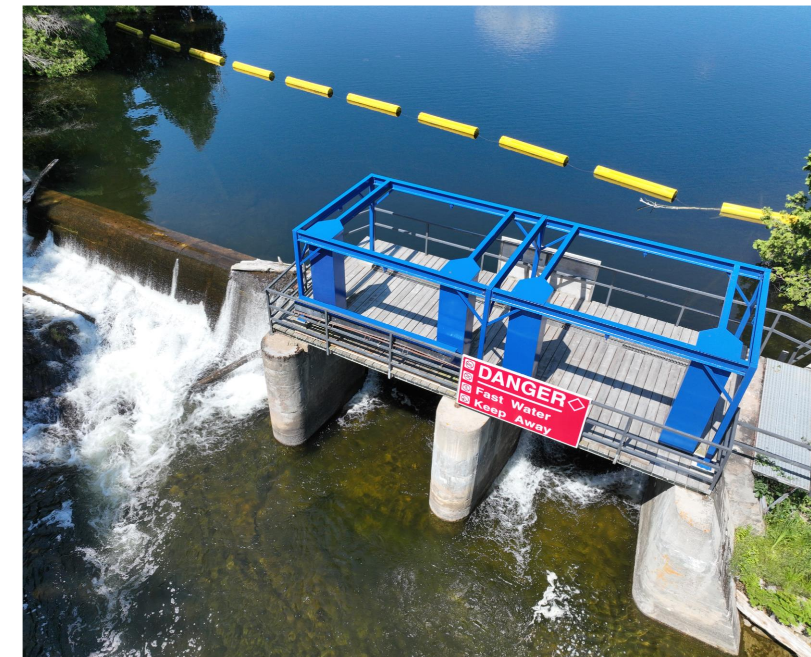
Main Kashwakamak Lake Dam Structure
